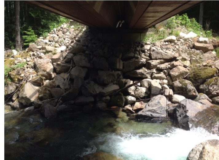
Right Bank Abutment when facing downstream
