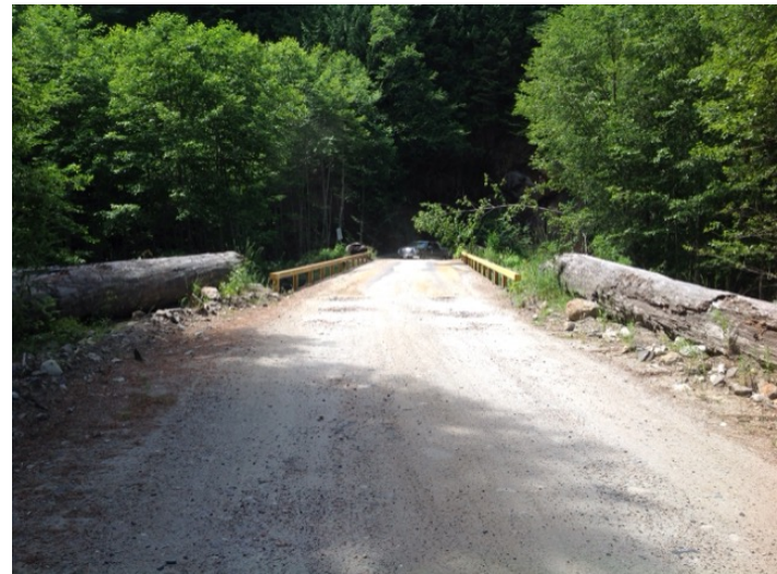
Approach from Right Bank when facing downstream
