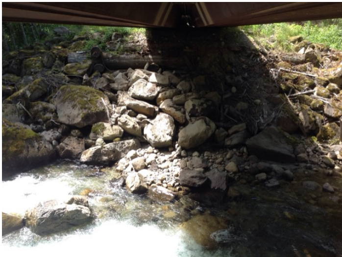
Left Bank Abutment when facing downstream
